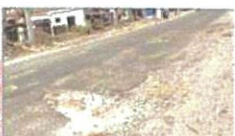
A VIEW OF ROAD IN BELI CHARANA AREA OF
