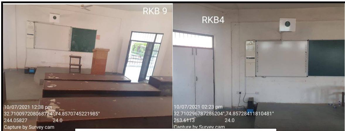
SMART CLASS ROOMS IN RADHAKRISHNAN BLOCK
