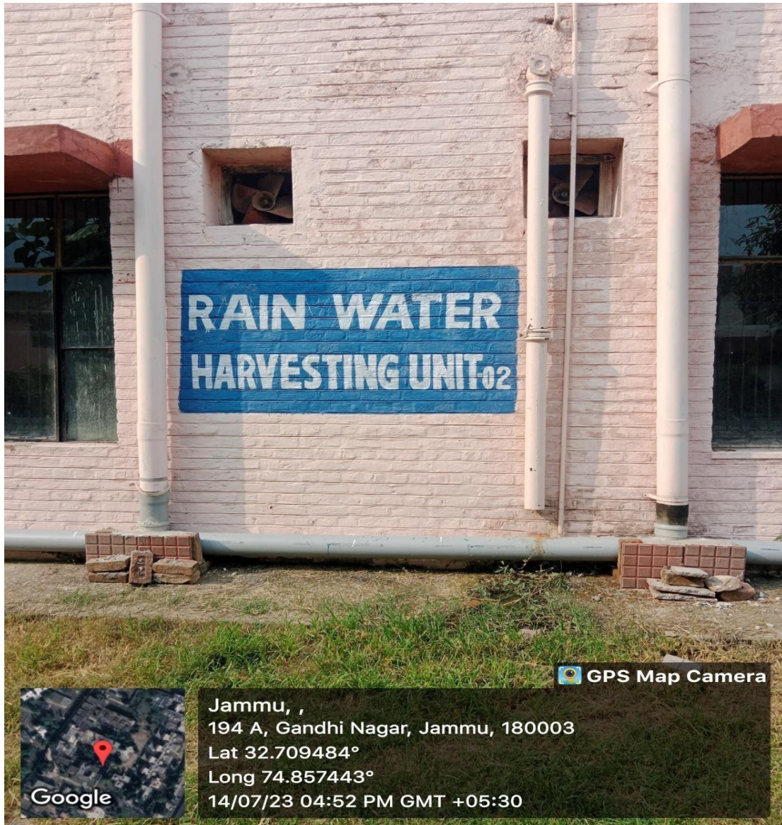
Rain Harvesting Unit-2 near Botanical Garden
