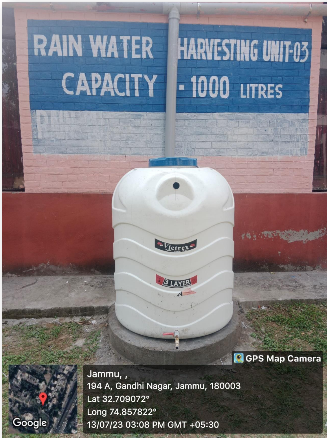
Rain Harvesting Unit- 3 near Library of the College
