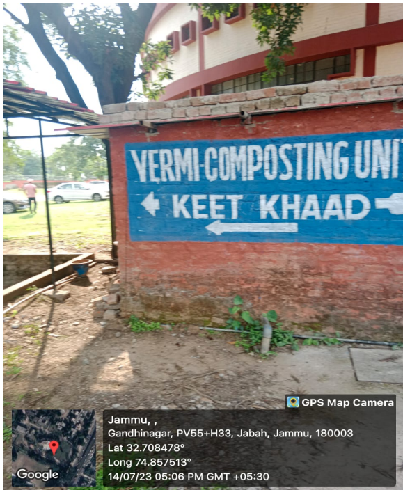
Vermi Composting Unit
