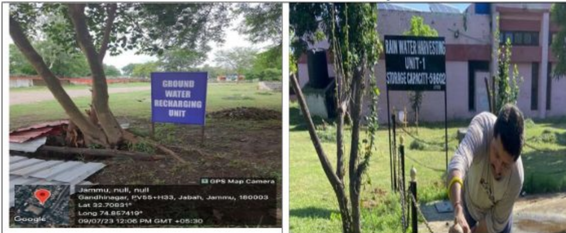
O1. Ground water recharging unit
