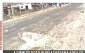
A VIEW OF ROAD IN BELI CHARANA AREA OF
